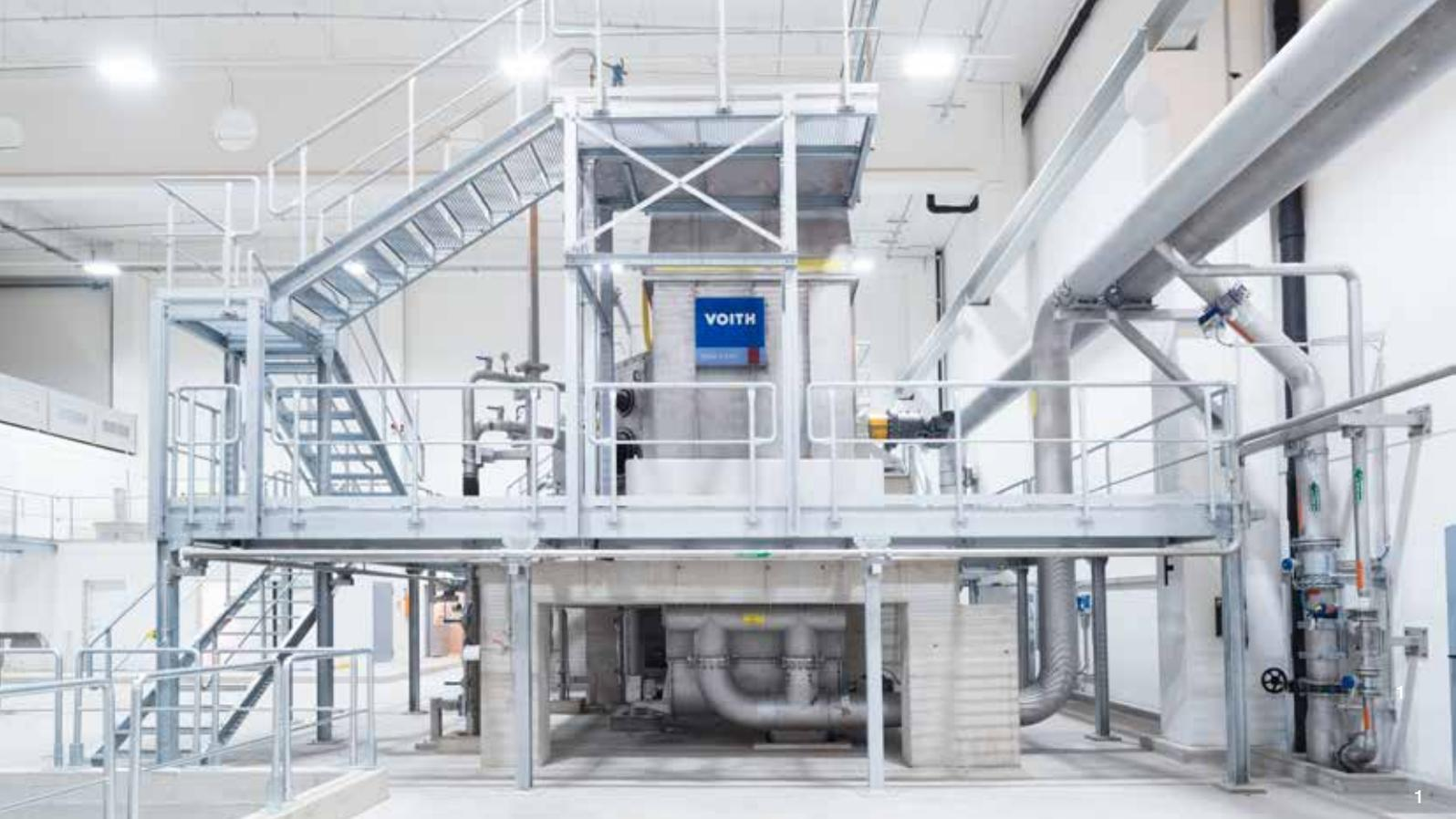
Continuous filtrate quality over a long period as well as low operation and maintenance costs are essential for a reliable and efficient dewatering process. However, fiber suspension thickening inside the vat can lead to mechanical stresses and damage to the discs. As a result, typical filters operate with limited inlet consistencies. This requires significant pumping of dilution water and the use of filters sized for a high volumetric load.
